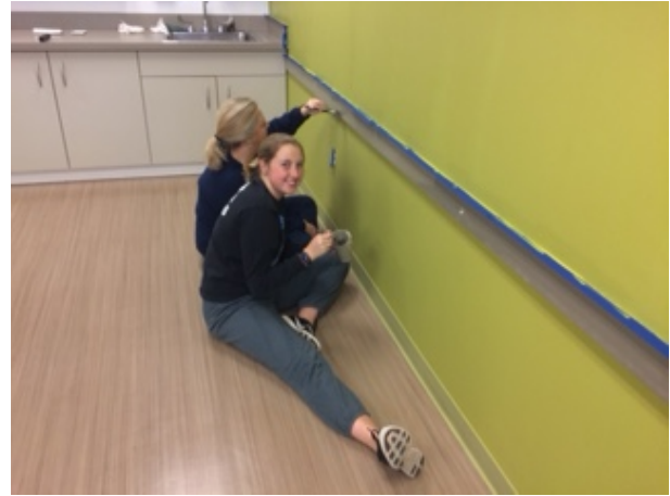
Volunteers paint the lower half of the wall
