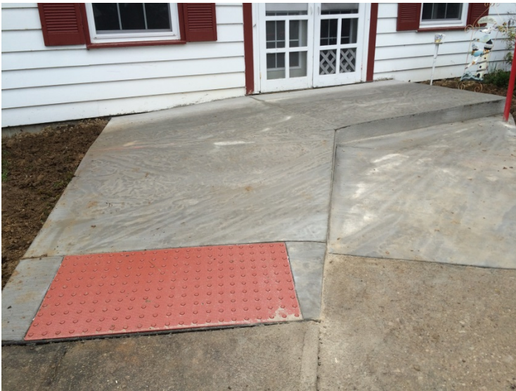
New concrete walkway and ramp outside Palda Cabin
