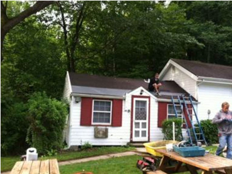
Roof repair project at Miller Cottage
