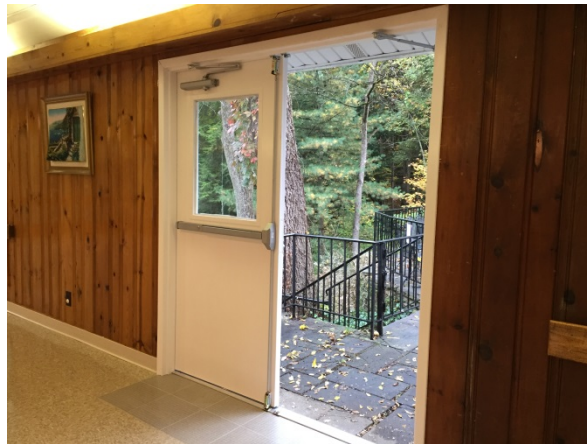
New double doors in Smith Lodge
